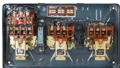
Interior View of MK2 FASD
