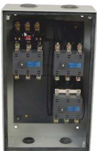
Interior View of ML SASD
